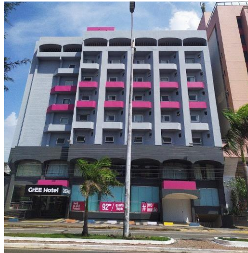
Figure 2 – Green Hotel facade
